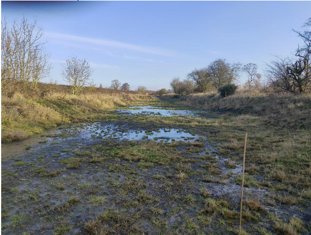
Photo Two – close up shot of the infill section to be excavated.
