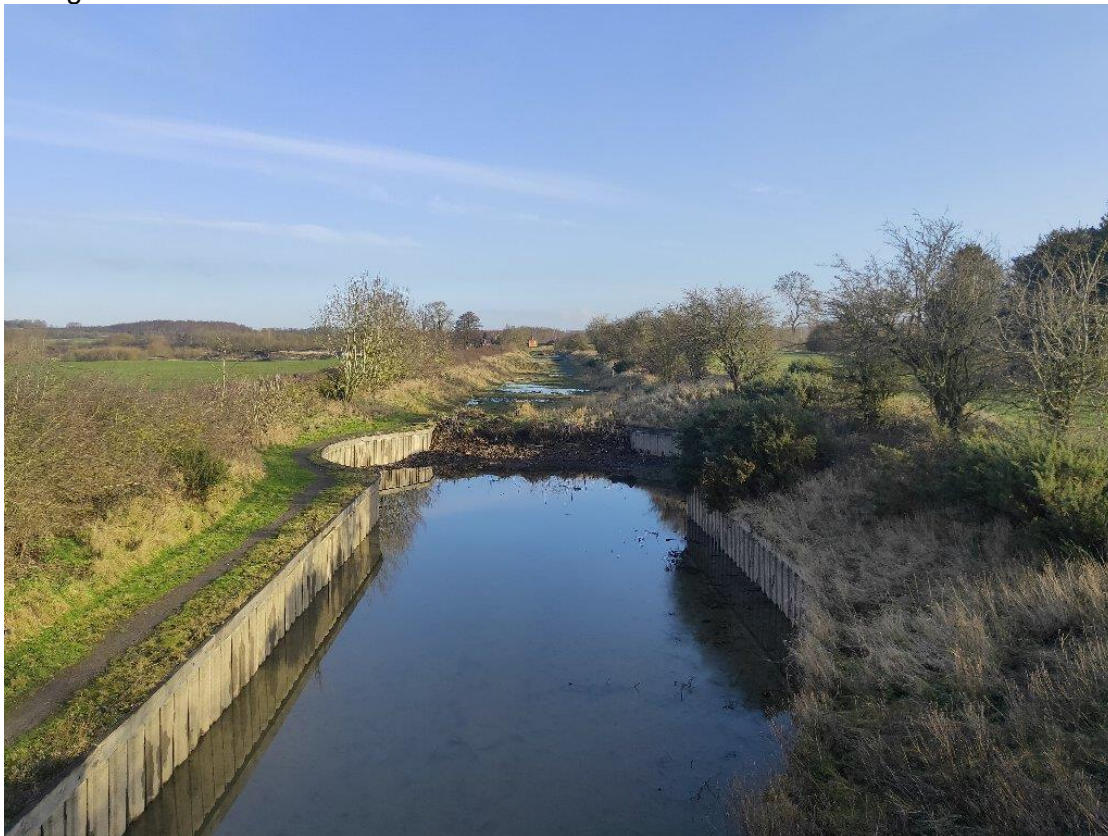
Photo One – view from Bridge 62, foreground shows the watered section and the background shows the infill section to be excavated.
